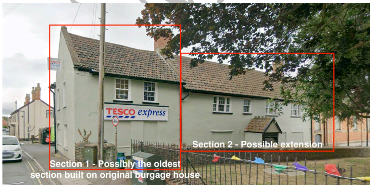
Figure 8 - Visible sections on the building - From Google Street Maps
